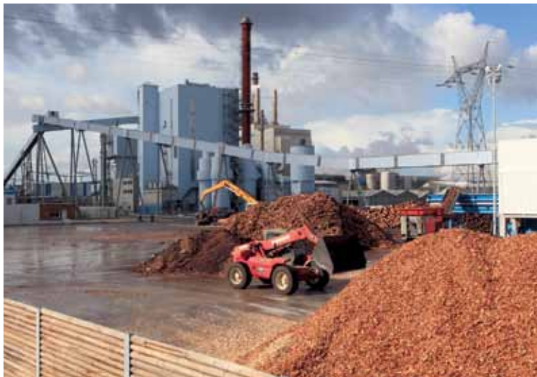
One of the largest biomass power plants in Central Europe is located in France and operated by Dalkia, one of Europe's largest energy service providers. The combined heat and power plant uses mainly bark and forest residues as fuel to produce 50 megawatts of electricity for the national grid and 74 megawatts of process steam for Smurfit Kappa's paper mill.
